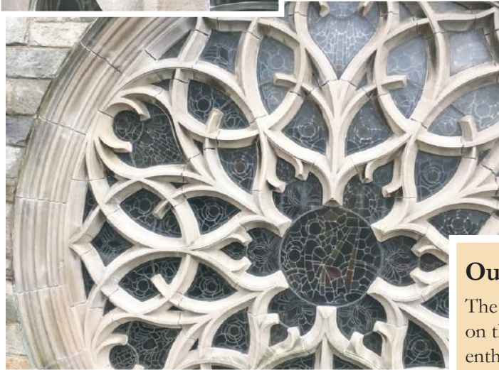
North window photographed before power wash and after grinding joints.
