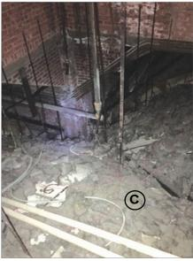
In the same picture above, the Church tower will need attention. At the top of the tower, there is a cross sitting on a four-sided copper roof. The pictures at left, taken inside the tower, show that there are signs of water damage below that copper roof (letter "B"); there is also an inner roof (letter "C") at the base of the tower that needs to be replaced. An inner drain pipe in the tower is clogged. We are awaiting a bid for this work.
