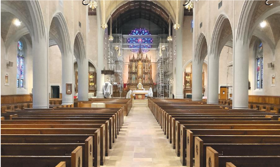
Our restored nave with new lighting, clean floors, and new kneelers
