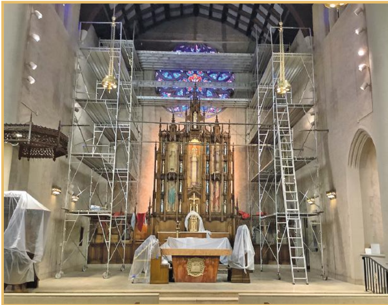
The sanctuary under restoration.
