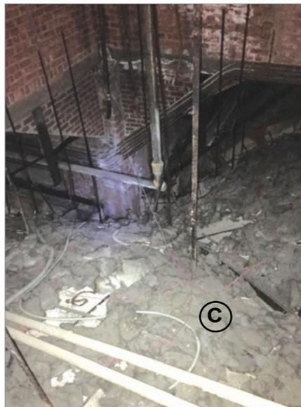
(2) In the same picture above, the Church tower will need attention. At the top of the tower, there is a cross sitting on a four-sided copper roof. The pictures at left, taken inside the tower, show that there are signs of water damage below that copper roof (letter “B”); there is also an inner roof (letter “C”) at the base of the tower that needs to be replaced. An inner drain pipe in the tower is clogged. We are awaiting a bid for this work.
