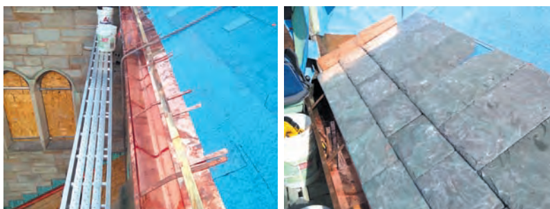
Roof materials include slate, tile, copper; work includes removal/replacement of roofing membranes, copper flashing, damaged slates, storm-damaged gutters, and restoring discolored features
